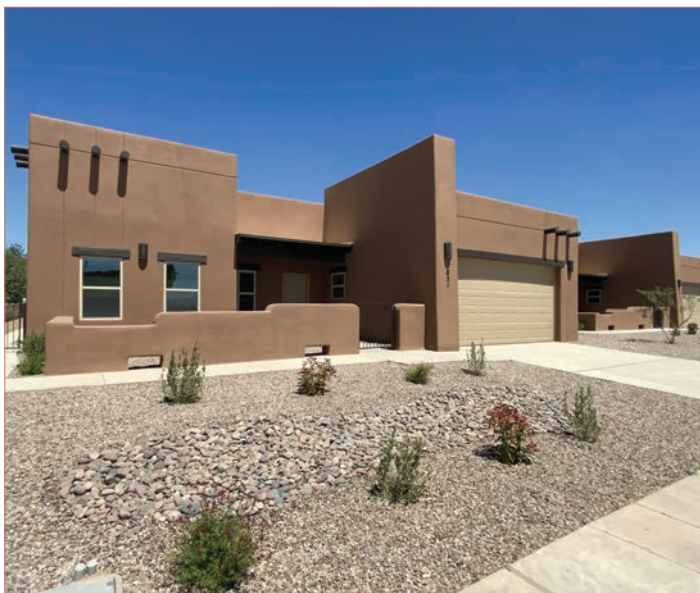
New home construction in District II.
