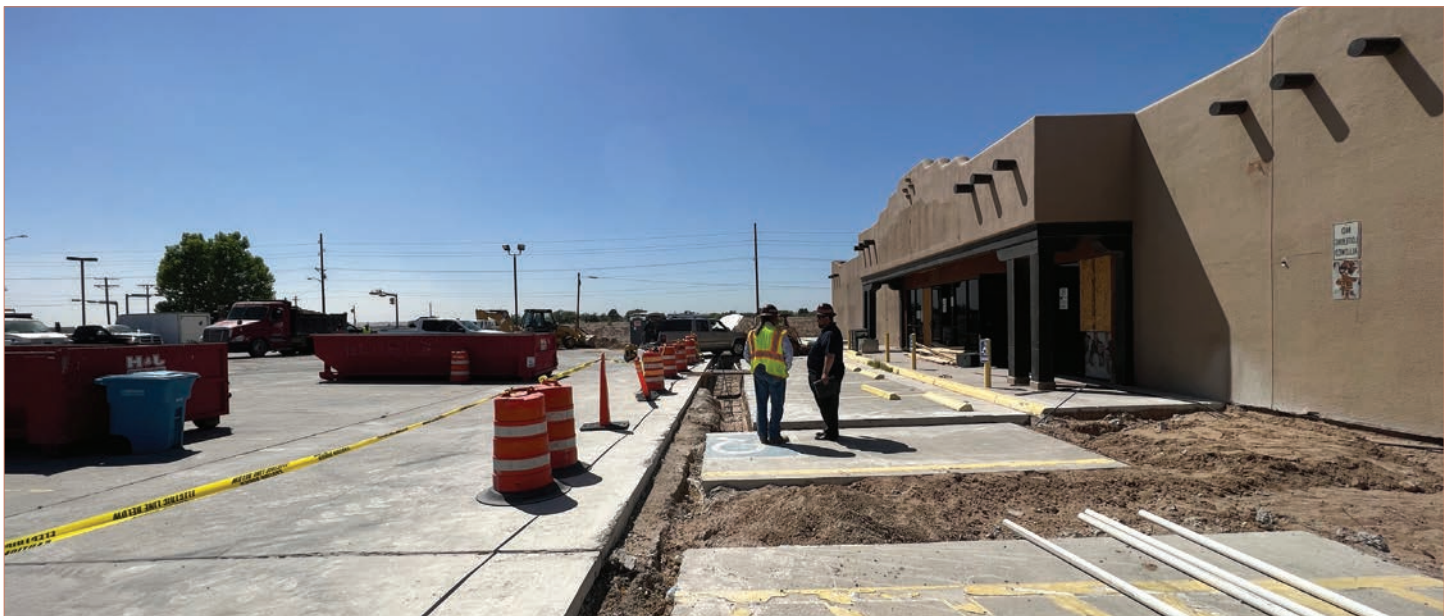
DPS new Tribal Communications Center
