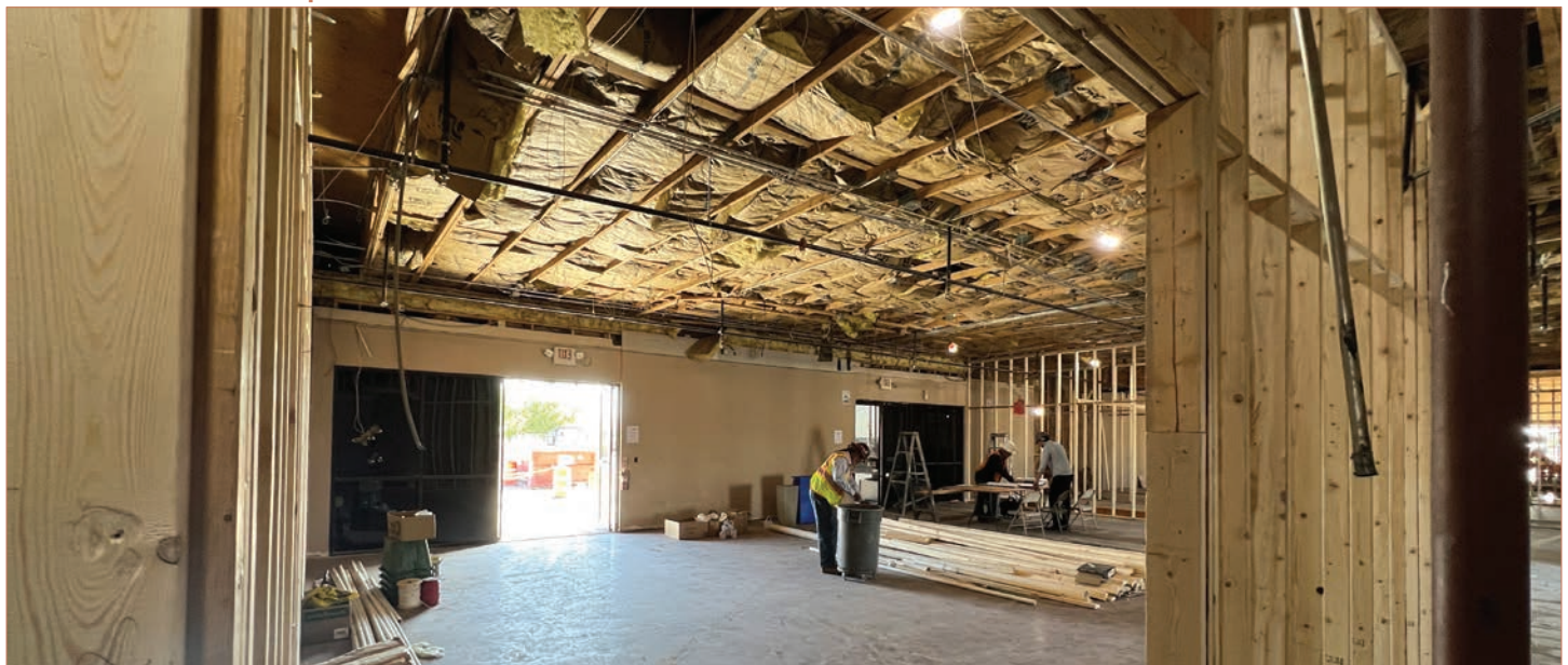
Construction of new Tribal Dispatch
